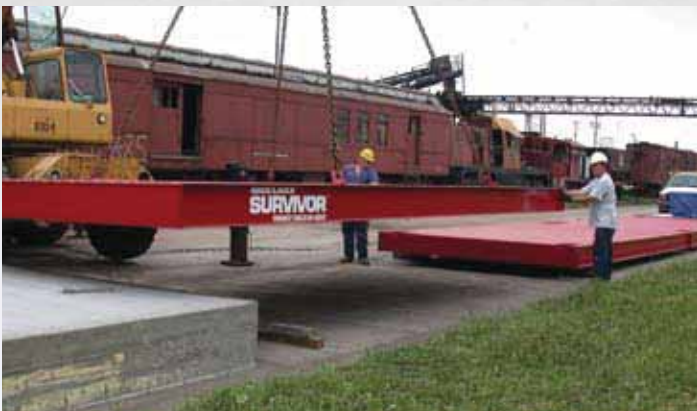
Module C is lowered into place.
